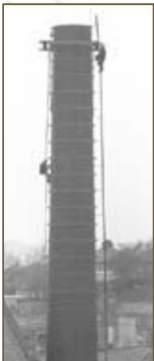
Calf Hall Chimney
